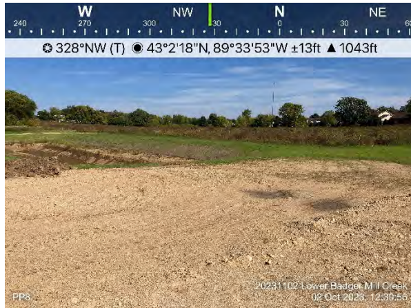
Photo #19 Photo point 8, view northwest from bridge
