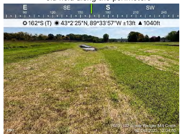
Photo #18 Photo point 7, view SSE along constructed swale for Lower Badger Mill Creek
