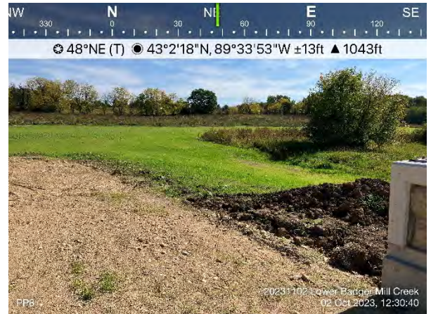
Photo #20 Photo point 8, view northeast from bridge
